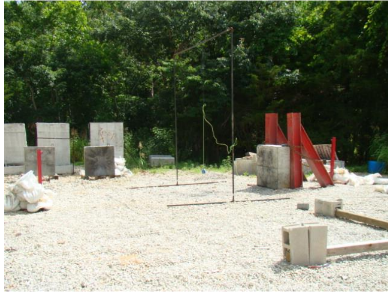
Figure 6.1 Barrier chained to supporting I-beams
