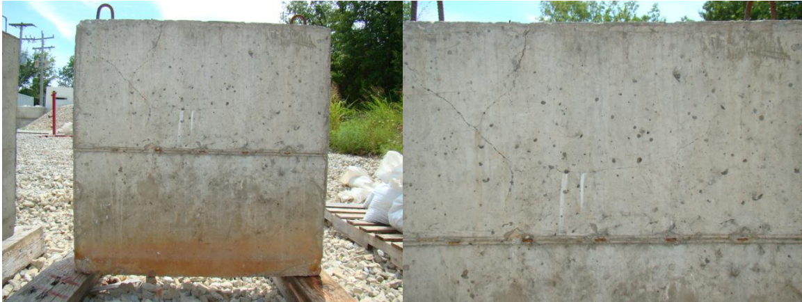
Solid concrete barrier
